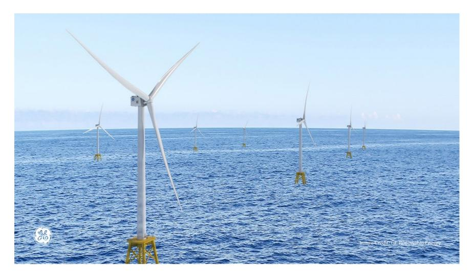
Featuring a traditional 3 blade 12 MW Offshore Wind Energy Generator (turbine) – Credit: GE Renewable Energy
