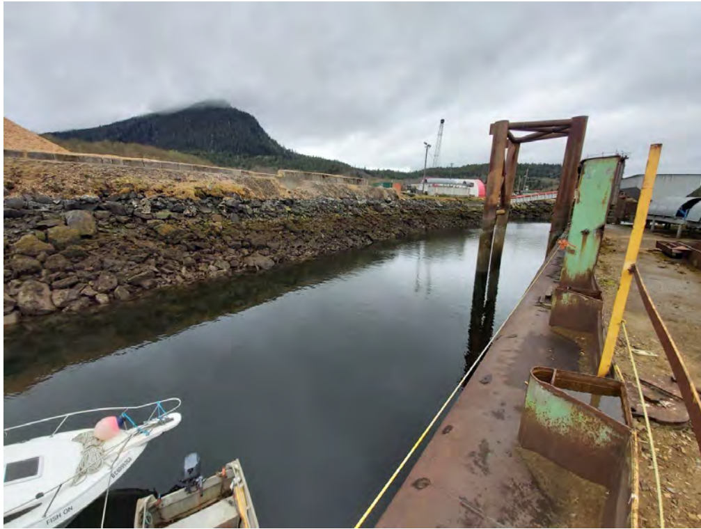
Figure 3. Photographs taken from middle of barge facing foreshore.
