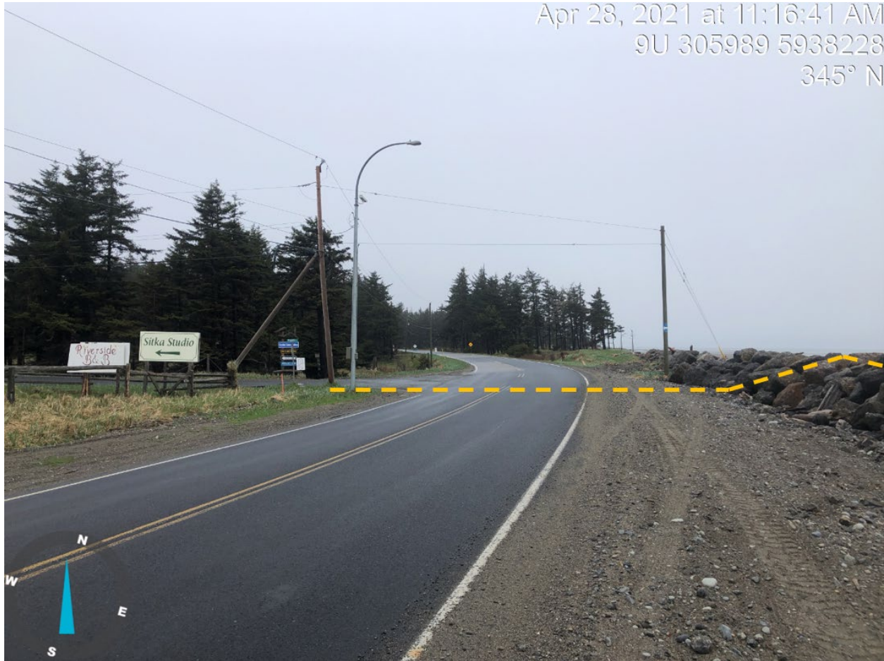
Photo 2 Cable alignment connecting to existing power pole in upland area of Tlell landing site.
