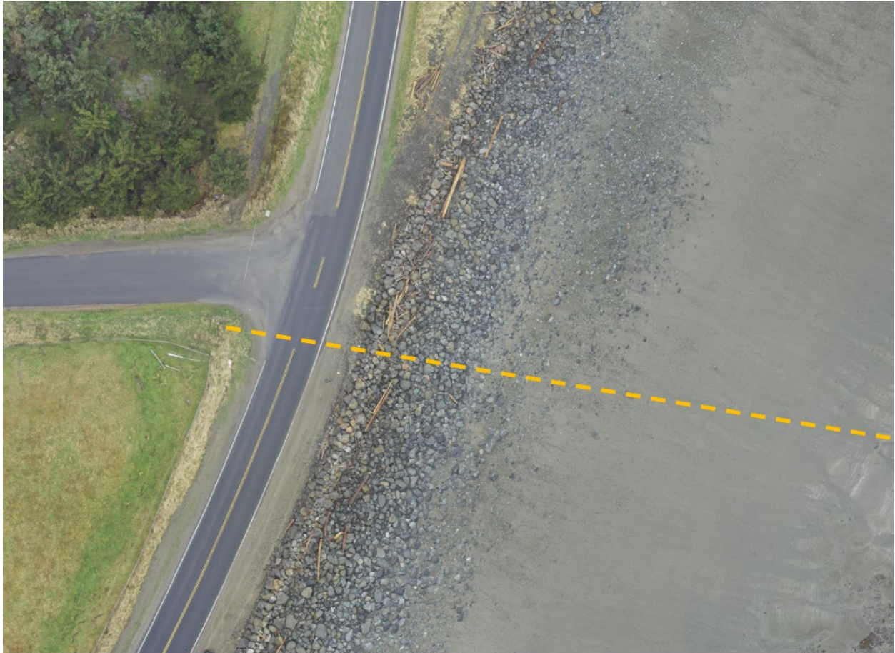
Photo 1 Overview of cable alignment at intersection of Yellowhead Highway and Wiggins Road.
