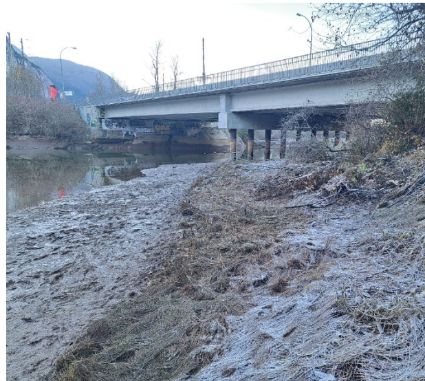
Photo 3: Looking at northern foreshore area from northern bank. November 24, 2023
